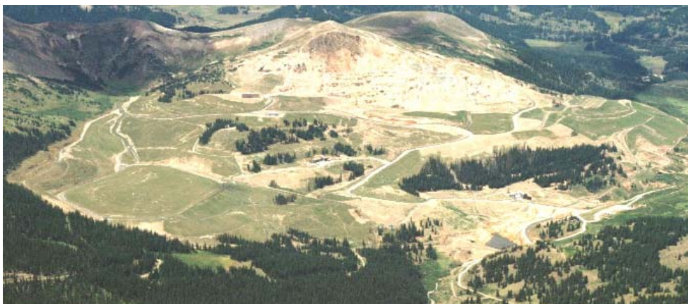
OU4 site-wide reclamation, completed in 2001, is designed to create stable ground surfaces and a vegetative cap so that clean water stays clean as it leaves the site.
