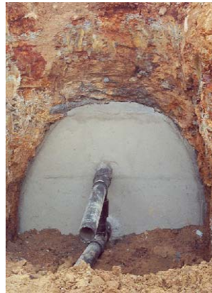
Crews plug the adit above. Left, the finished wall at the "Little Stella Adit."
